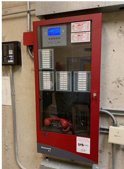
Panel replacement and related update work
