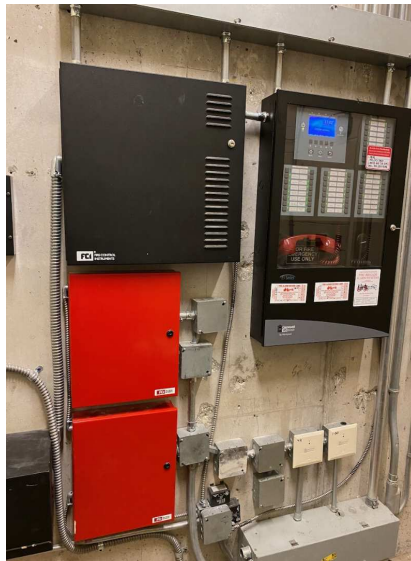
Panel replacement and related update work
