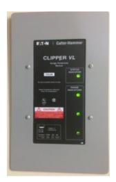
If one or more of the lights is not working there may be a serious problem within the surge protector. Failure of the surge protector may result in serious damage to the electrical system and electrical appliances and devises.
